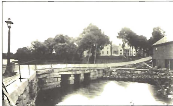
Site of former lumber and grain mill on Main Street.
